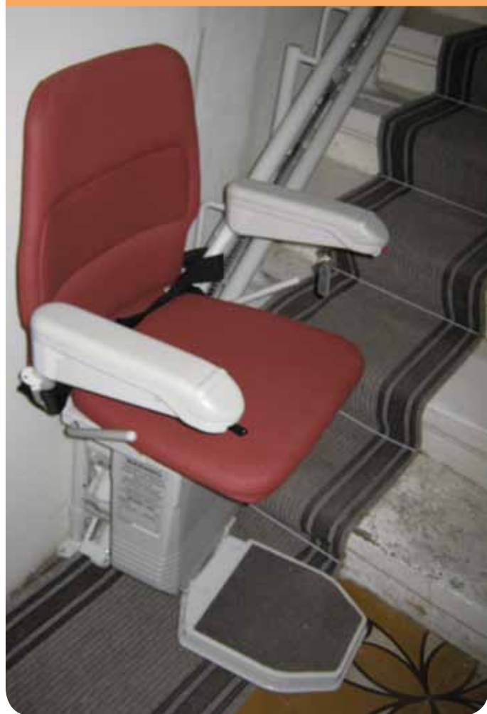
Stair lift installat f'residenza f'Birkirkara
