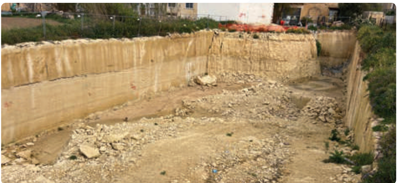
Excavation Works at Tank Street, Siġġiewi
