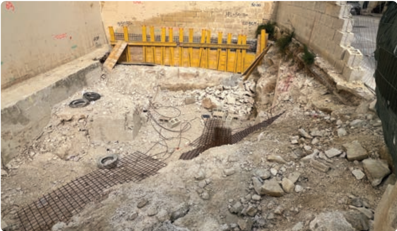
Excavation Works at S. Imbroll Street, Paola
