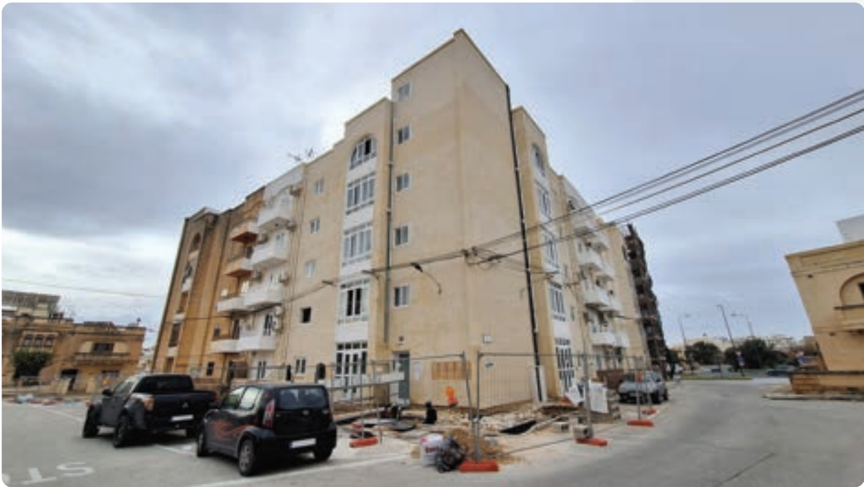
Block L, Żabbar – Deep Energy Renovation Project
