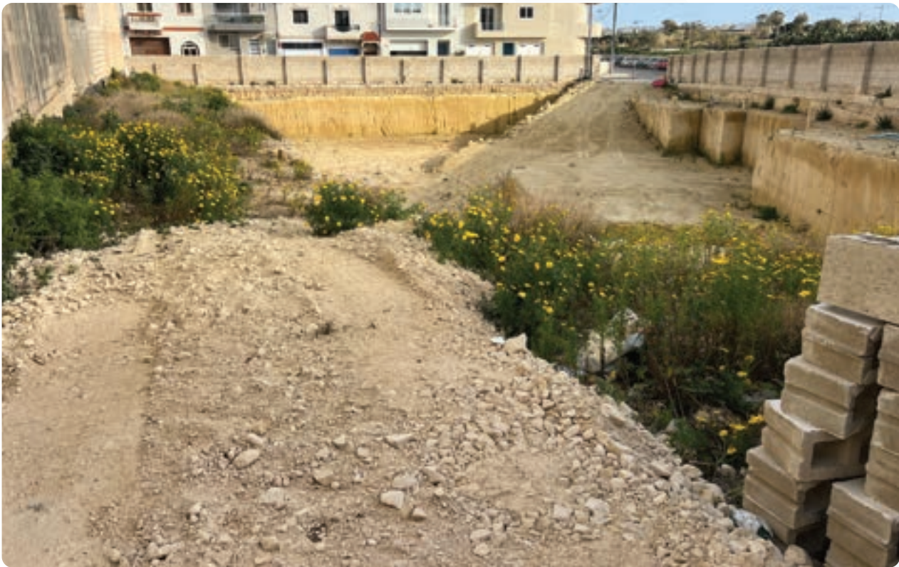
Excavation Works at Serafin Tanti Street, Żebbuġ
