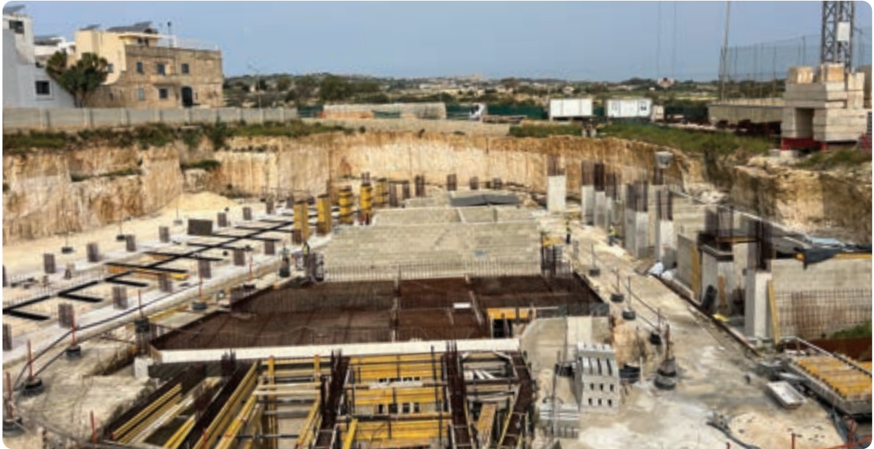
Foundation Works at Wied Hesri Complex, Siġġiewi
