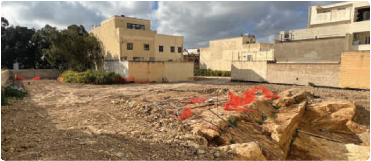
Excavation Works at Karwija Street, Kirkop
